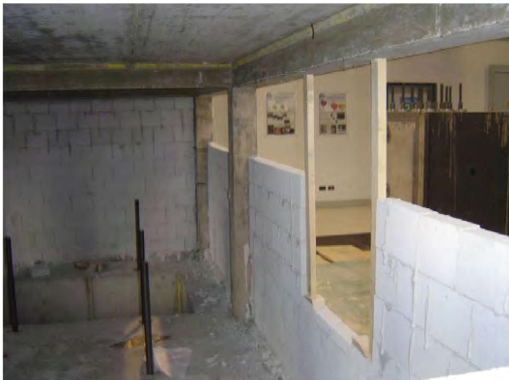
Figure 6–4 The specimen infill panels are made of cellular concrete Gasbeton RDB, thickness 50mm
